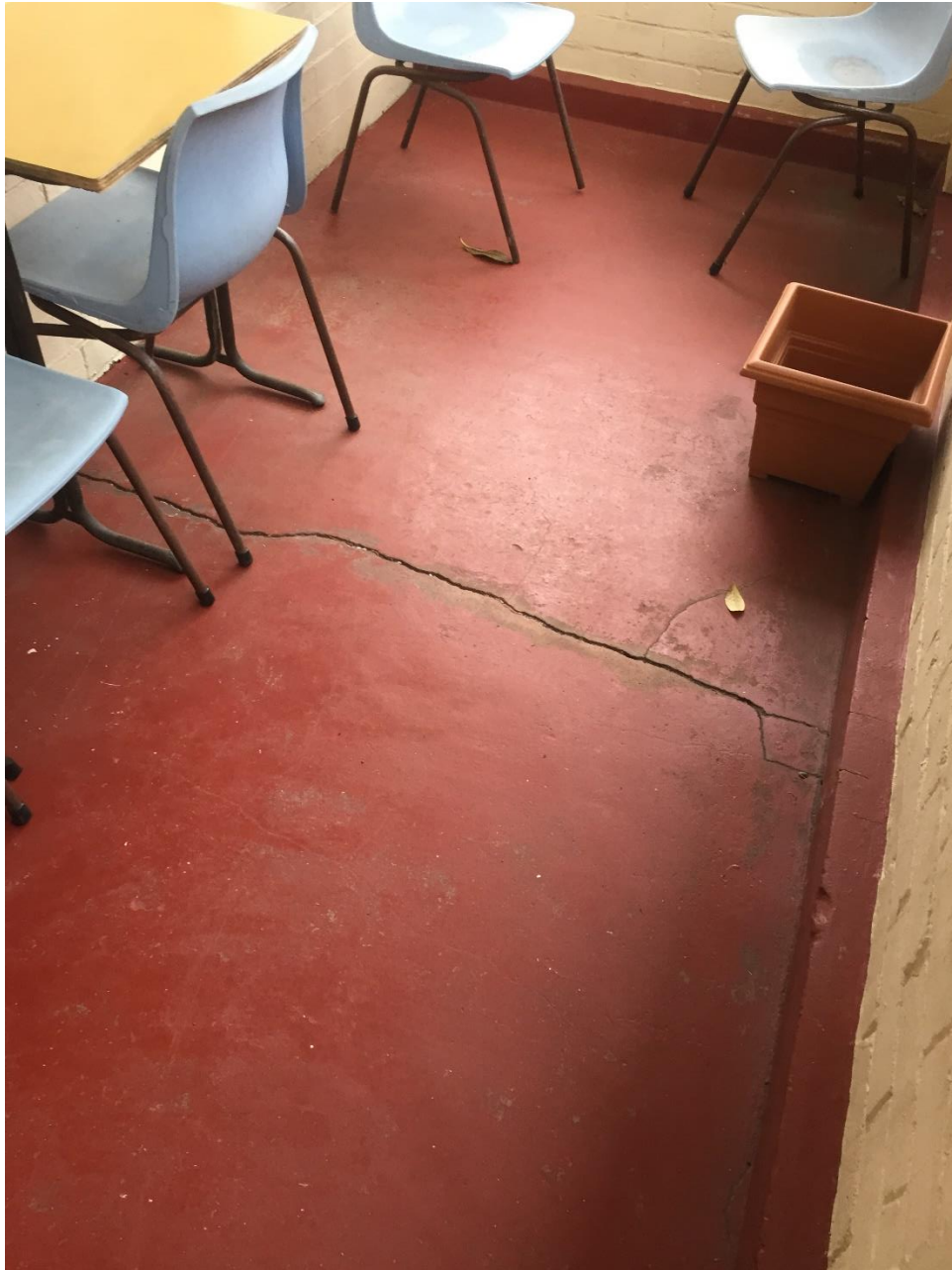
Figure 16 - Front verandah painted concrete detail. Showing cracking due to subsidence of sub floor fill. The later verandah enclosure is seen on the right.
