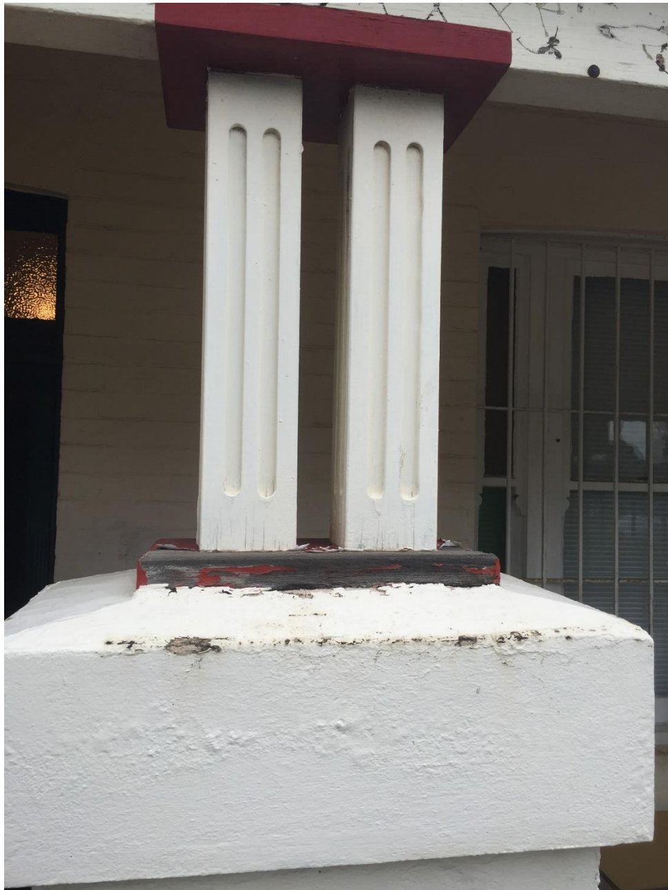
Figure 17 - Modern replacement verandah supports with routed detailing. There is no evidence of the original details, however the layout and surviving details on the side of the verandah suggest bracketed posts which were typical of the period when the former house was built.
