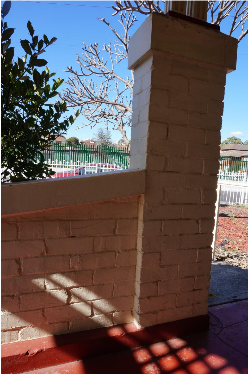
Figure 15 - later Brick verandah enclosure and piers. The front of the building was modified at some point in its history to remove the original Federation detailing and replace it with this Inter War style details. The brickwork does not match the rest of the front façade which is carefully tuck pointed and the character is at odds with the original character of the former house.
